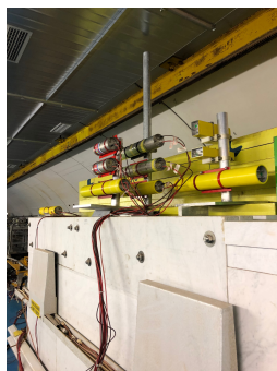
Figure 5: ESS and LHC type chambers installed at HiRad-Mat.
