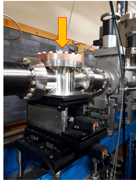
Figure 7: EPU-PBPM installation at the front-end of BL10A.
