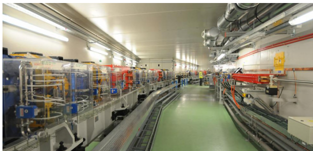
Figure 1: View of the Accelerators’ tunnel; on the left the storage ring, and on the right the booster. Picture taken on the 8 th of September 2009 (J. Klorá).
