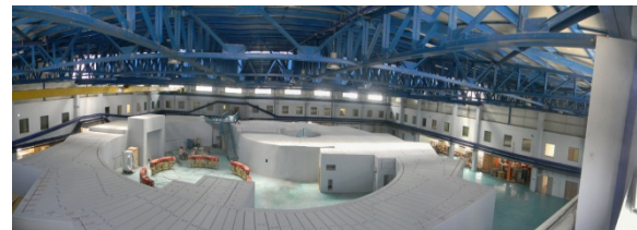
Figure 1: SESAME radiation shielding wall.
