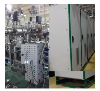
Figure 4: RFQ LCS junction boxes (on the left) and cubicles (on the right).
