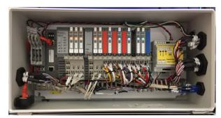
Figure 3: EPS remote I/O box module layout.
