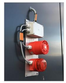
Figure 7: Alarm plate installed in the facade of the HCB.
