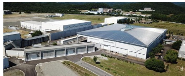
Figure 2: NewSUBARU building and new annex building for the new linac.
