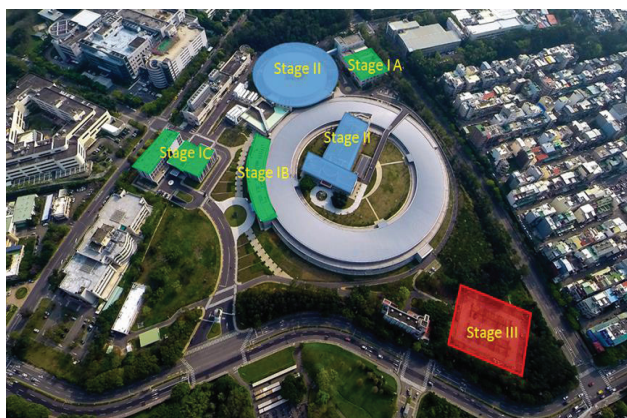
Figure 3: Areas of three stage of the installation of solar PVs.
