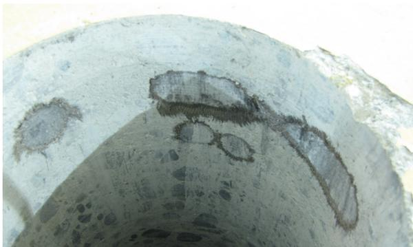
Figure 3: A coring close to the beam path showing steel re-enforcement bars with iron filings adhering to the rebar edges due to remanent magnetization.
