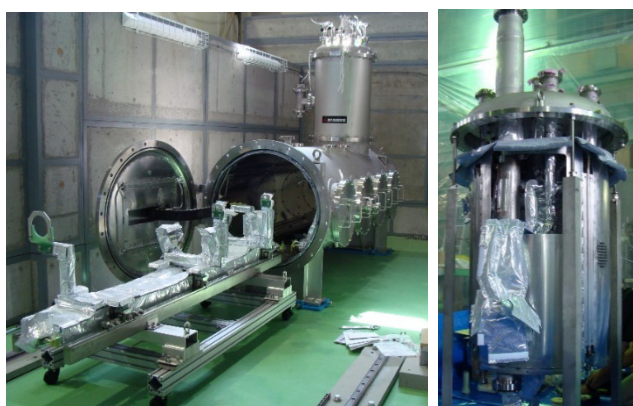
Figure 1: (left) Installed horizontal test cryostat. (right) Inside cold box.
