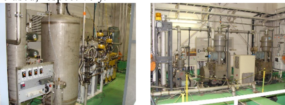
Figure 4: (left) He gas recirculation system. (right) He pumping system.
