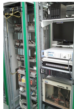
Figure 3: RFQ Racks preparation for power test.
