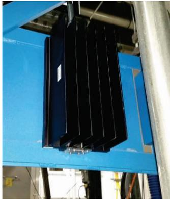
Figure 5: Air-cooled load, installed in DTL-5.
