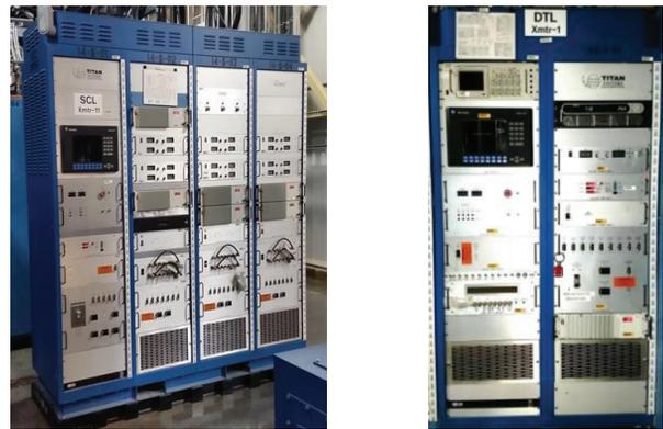
Figure 1: Typical SCL and DTL/CCL Transmitter Racks.
