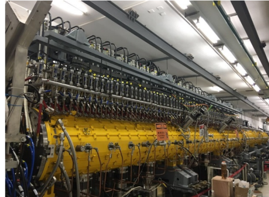
Figure 1: CSNS DTL-1 in the linac tunnel.
