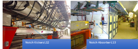
Figure 1: Hor. Notching kickers and absorber.
