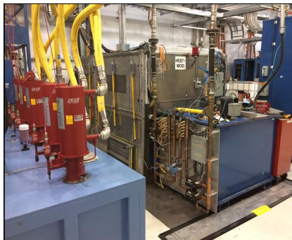
Figure 4: Prototype PPU HVCM during a heat run.
