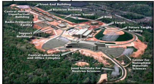
Figure 1: Overview of the SNS in Oak Ridge, Tennessee. Major facility buildings are superimposed on an aerial photograph of the construction site.
