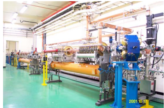
Figure 1: A photo of Test Linac tunnel.
