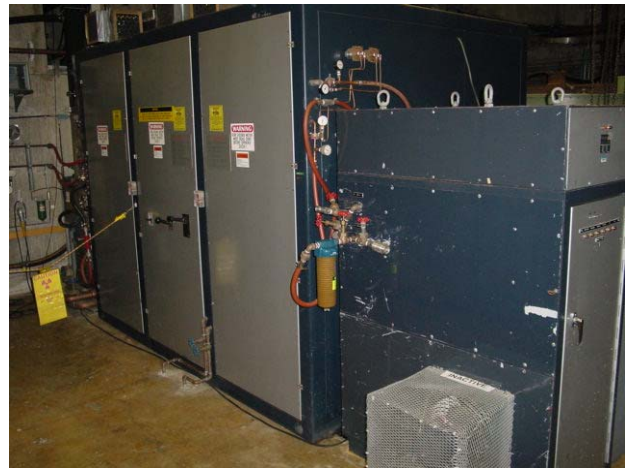
Figure 3: Klystron modulator.
