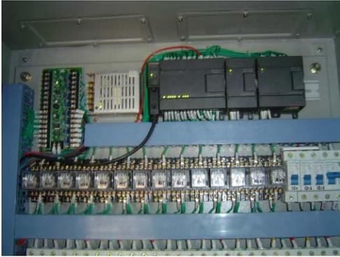
Figure 6: Siemens 200 PLC Controlling of 80kW cooling water system.
