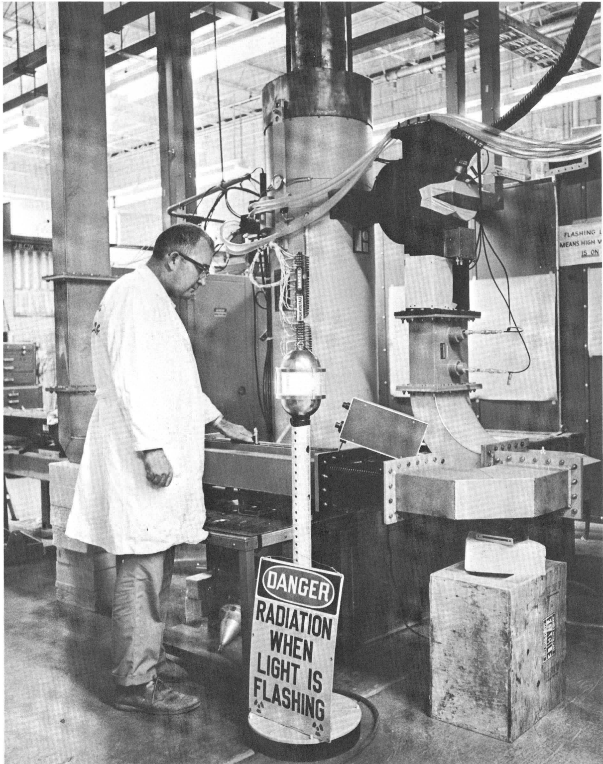
Figure 2 — The first Litton klystron received at IASL mounted in its magnet. The modulator is contained in the rectangular oil tank resting on the floor.
