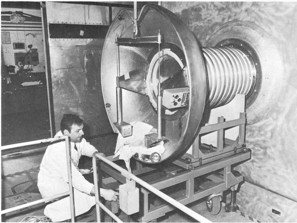
Fig. 3 Demounting of accelerating tube.
