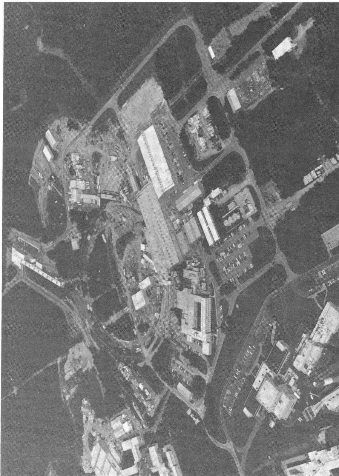
Fig. 1. Aerial view of the AGS Complex showing the Linac Complex on the far side of the ring.
