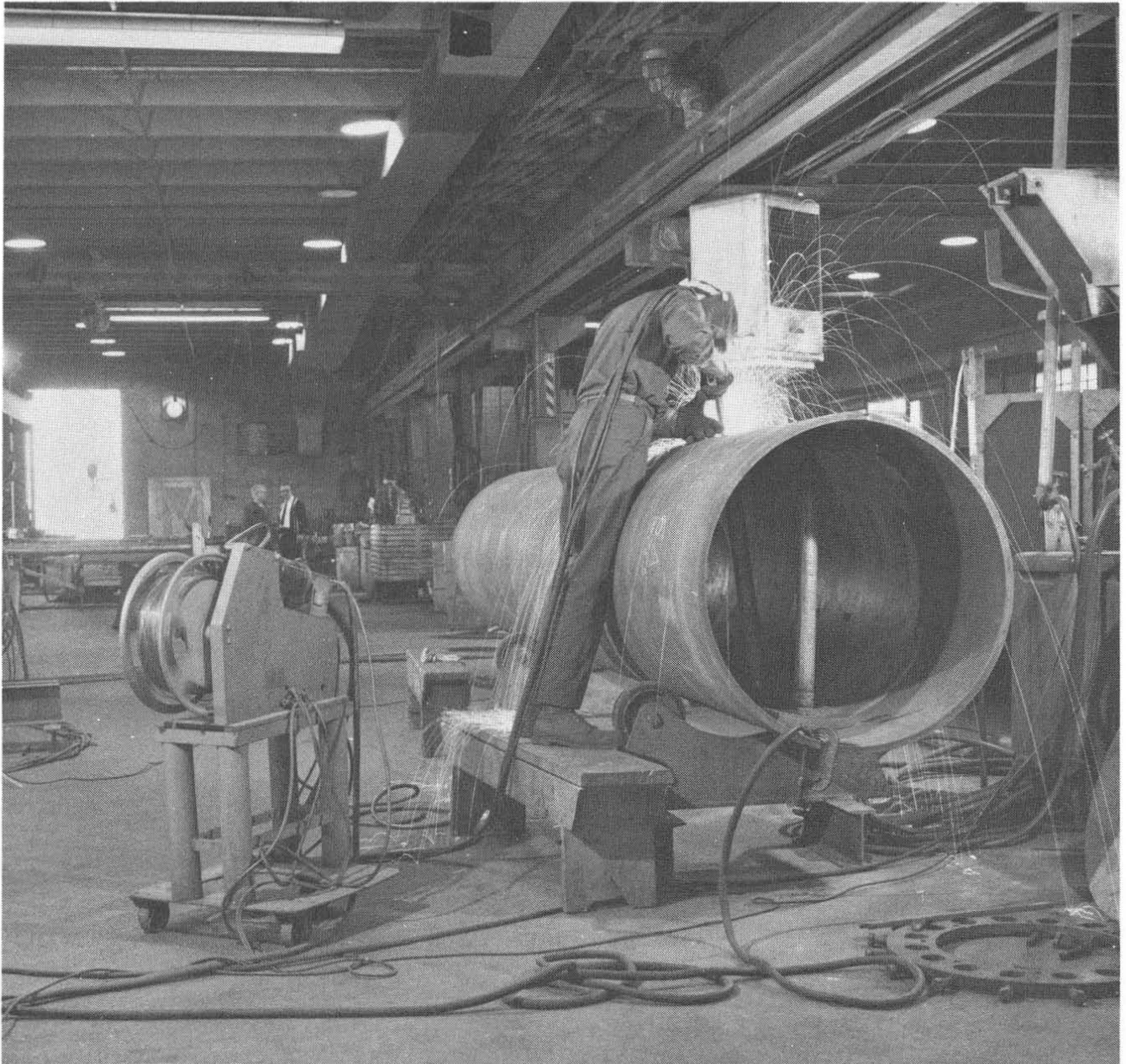
Fig. 5. Steel seam being welded.
