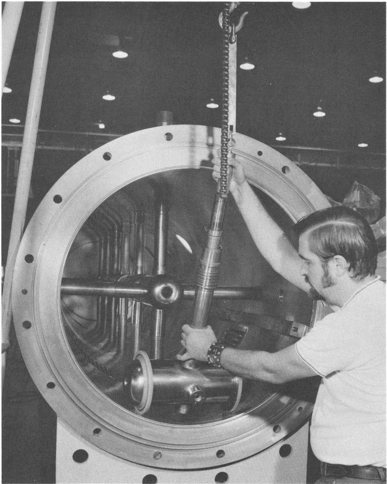
Fig. 13. Drift-tube installation.
