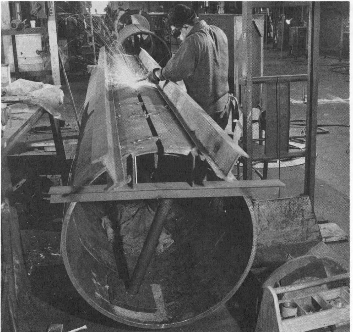
Fig. 3. Tack welding seam prior to cutting "J" groove.
