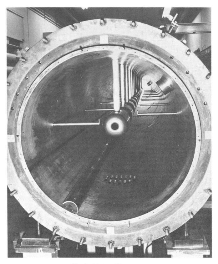
Fig. 1. Interior of linac cavity.
