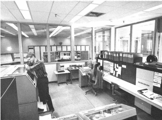
Fig. 11 Central control computer.
