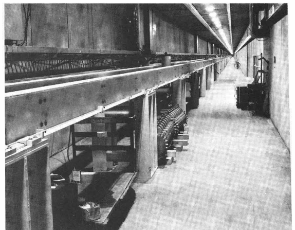
Fig. 8 805 MHz tank support structure
