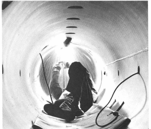
Fig. 6 Interior steel weld 201 MHz tank section joint
