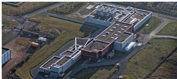
Figure 7: Completion of the SPIRAL2 building (October 2014). The beam axis is 8 meters underground.
