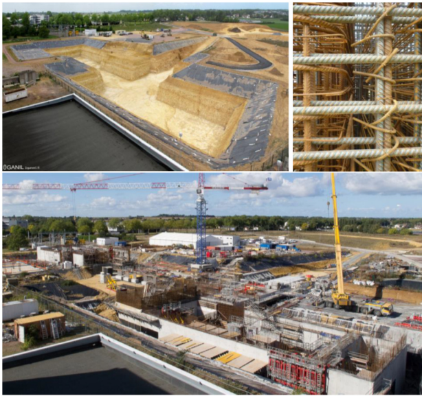
Figure 6: views of the construction site under way.
