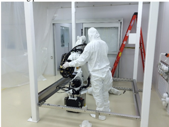
Figure 2: Installation of the robot and frame.
