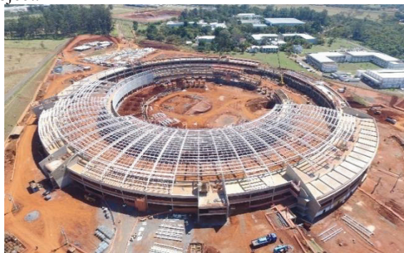
Figure 1: Sirius' construction status in August, 2016.
