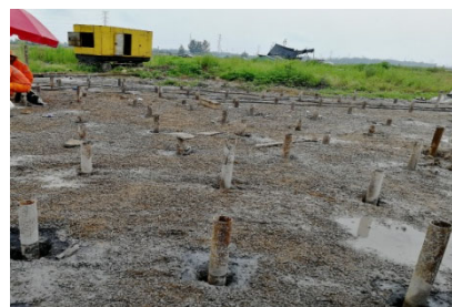
Figure 2: The prototype #4 slab: after grouting.
