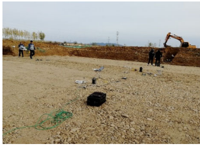
Figure 3: Graded sand and stone layer of slab #1.
