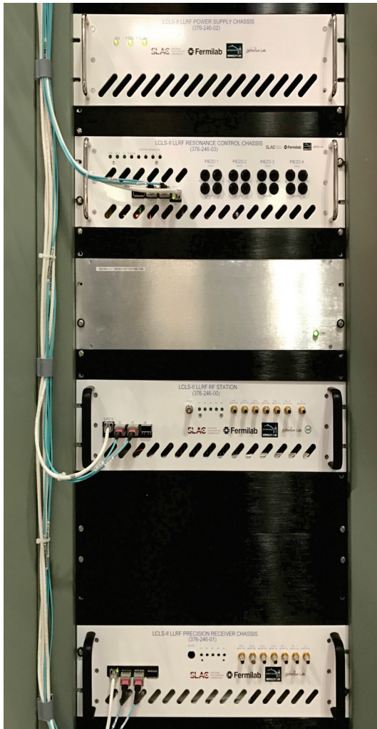
Figure 10: LLRF Testing at the FNAL CMTS.
