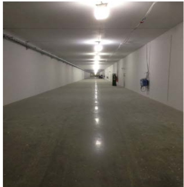
Figure 11: View of the ESS accelerator tunnel. The tunnel is 5 m wide by 3.5 m high
