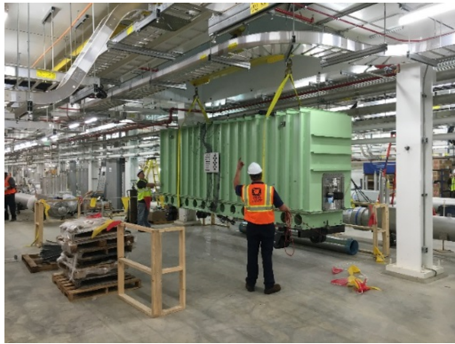
Figure 11: First FRIB \beta=0.085 cryomodule moved into linac tunnel for final installation.
