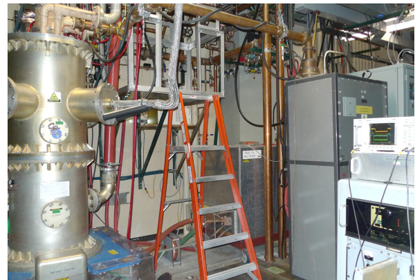
Figure 1: Legacy triode and tetrode RF amplifiers.
