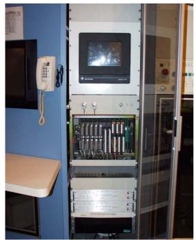
Figure 5: PLC and fast rf interlock.
