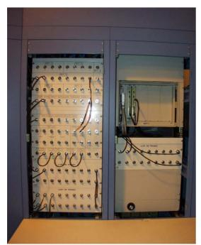
Figure 3: Low-level rf patchbay.
