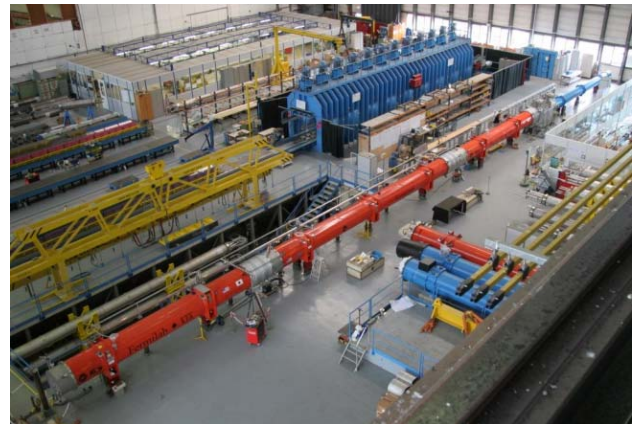
Figure 6. LHC Low- \beta triplet assembled at CERN before installation in the LHC tunnel.
