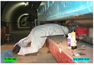
Figure 2: A Technician working on an installed dipole
