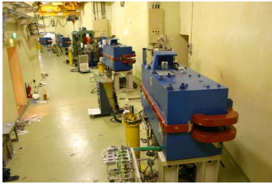
Figure 4: Old quadrupoles and beam ducts were completely removed from the straight sections.
