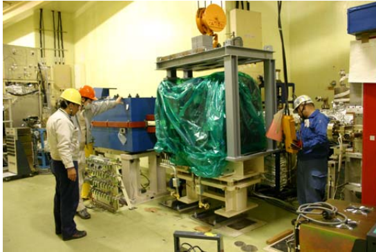
Figure 5: Installation of the new quadrupoles.
