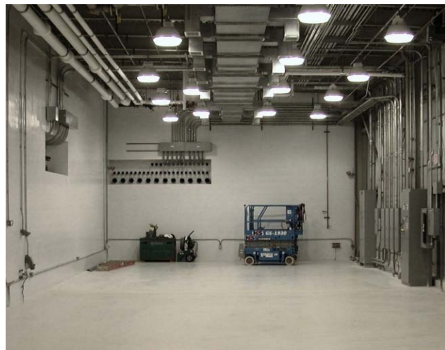
Figure 4: HEBT Service Building at Beneficial Occupancy – Apr '03.
