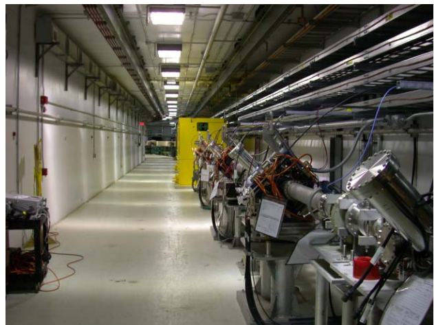
Figure 3: HEBT Beamline Installation – Apr '05.
