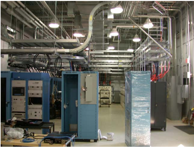
Figure 5: HEBT Service Building Installation – Apr '05.
