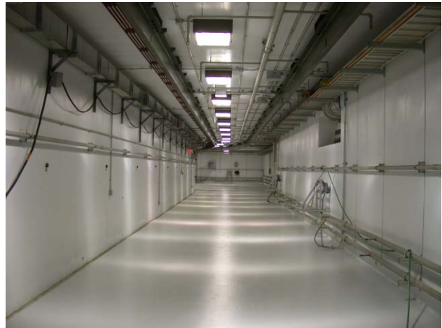
Figure 2: HEBT Tunnel at Beneficial Occupancy – Apr '03
