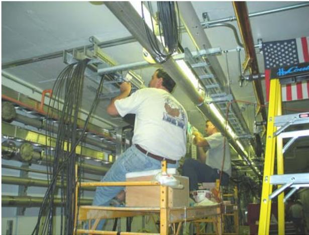
Figure 3: Installation of the electrical beamline interface.
