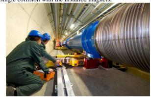
Figure 1: Transfer of a main dipole magnet on the support jacks.
