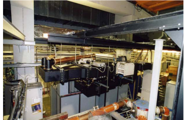
Figure 2: The switchless combiner.
