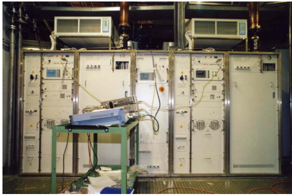
Figure 1: The RF power amplifier.
