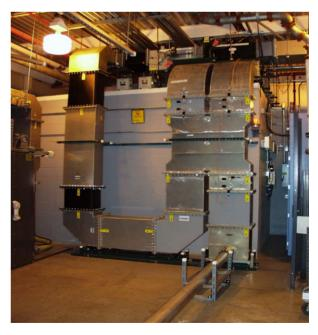
Figure 4: Photo of waveguide system showing 3-dB hybrid and 300-kW reject load installed on test stand bunker.
