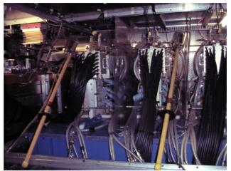
Figure 3: IGBT switching assemblies
