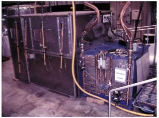
Figure 4: 15 MW output converter-modulator
