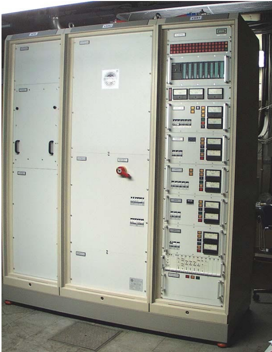
Figure 6: The first of three 100 kW amplifier delivered in December 1998. Left RF part, middle HV rack, right control rack
