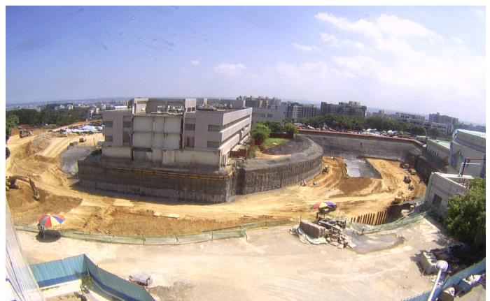
Figure 1: TPS construction site in Sep 2010.
