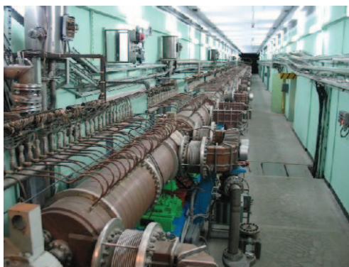
Figure 1: DAW accelerating structure in the INR linac.
