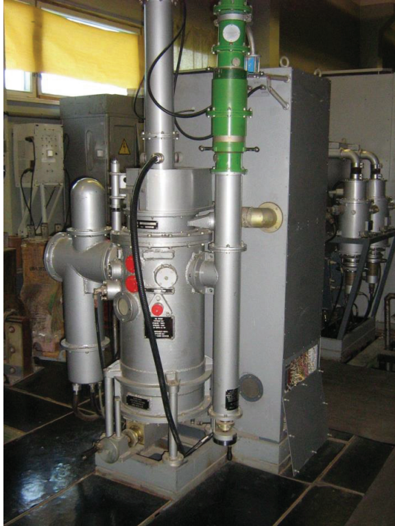
Figure 3: Intermediate power RF amplifier.
