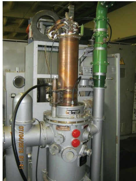
Figure 8: Intermediate power amplifier after revision.
