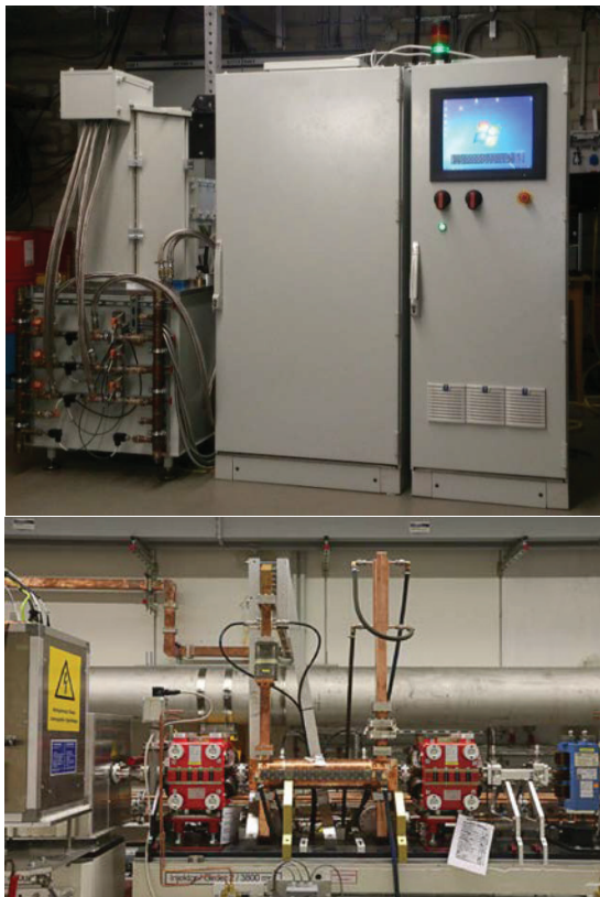
Figure 15: HPRF INJ and TDS structure INJ.
